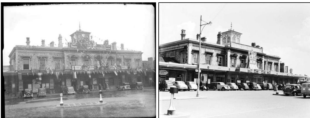
Fig 26: Reading General Station decorated for VE Day and the Coronation of Elizabeth II
