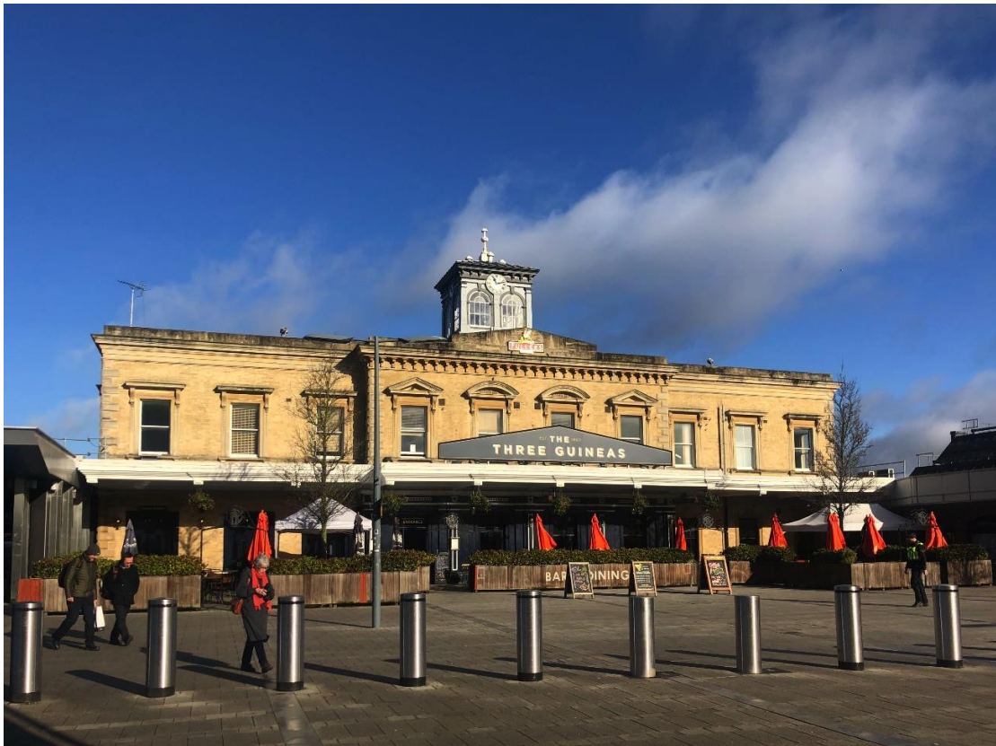
Fig 22: Main Building of Reading General Station
